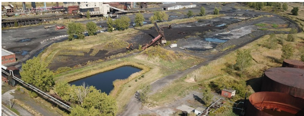
Photo 4-9: Looking Northeast at the coal yard before regrading and before removal of the stacker reclaimer (center of photo).
