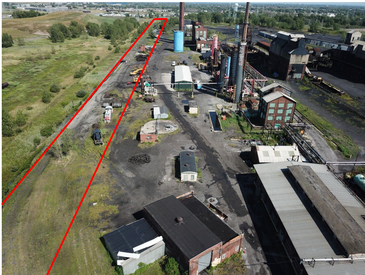
Photo 4-2: Looking east. August 2020. The redline approximates the northern, southern, and eastern limits of AOI1.
