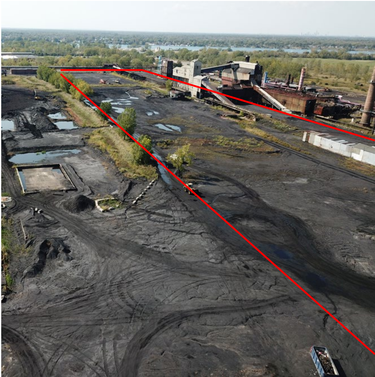
Photo 4-6: Looking Northwest Across the Coke Yard. The coal handling and coal charging buildings in the photograph were demolished in 2021
