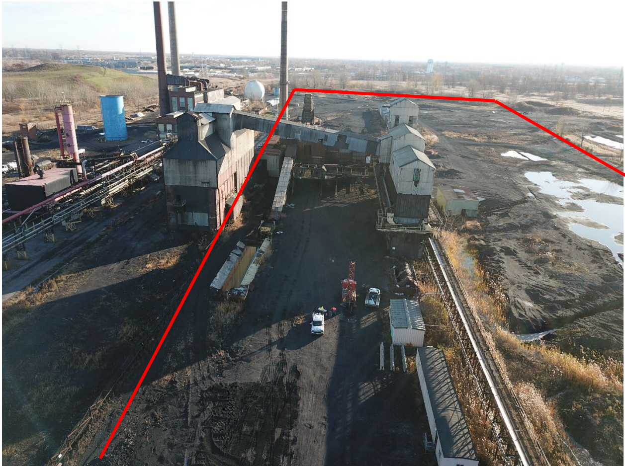
Photo 4-7: View Looking East Across Former Coke Rail Loading Yard (Northern Section of Coke Yard) in 2020.
