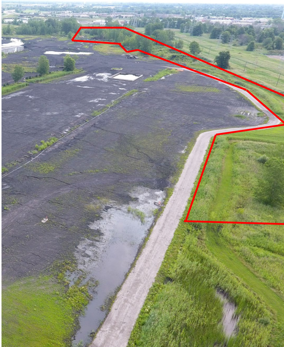
Photo 4-11: Looking east over the South Drainage AOI. Sedimentation Pool #001 is in the foreground of the photograph.
