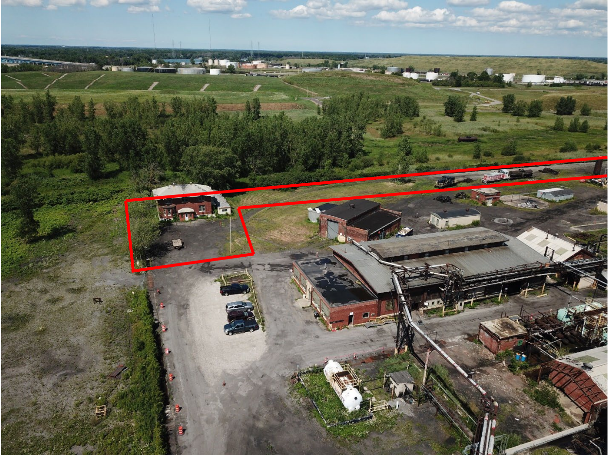
Photo 4-1: August 2020. Looking North. The redline approximates the west end of the North Rail Corridor (AO11).
