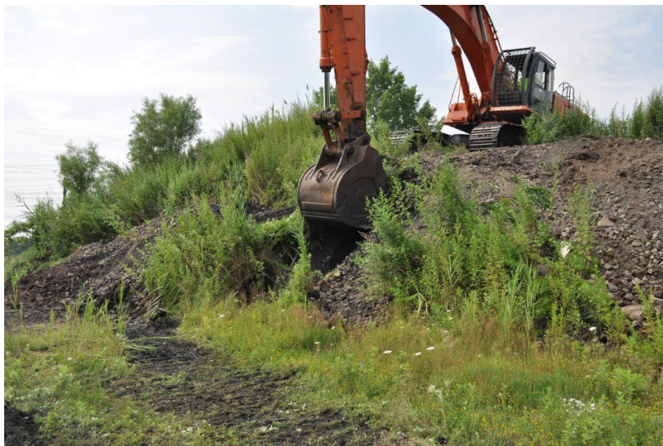
Photograph 4-11 (closeup) – Fill piles at the eastern end of the South Ditch.
